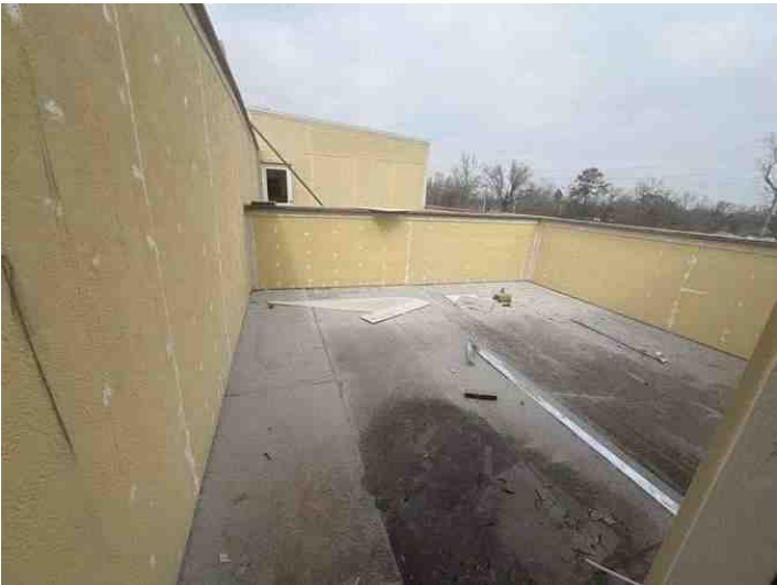
Subject Roof Top Patio
