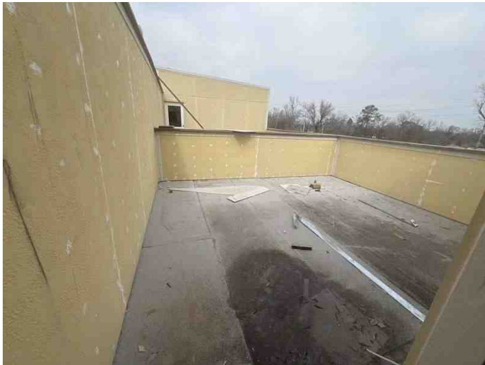
Subject Roof Top Patio
